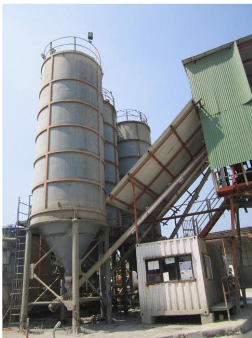
Figure 1 Steel Silo at RMC, Ernakulam
