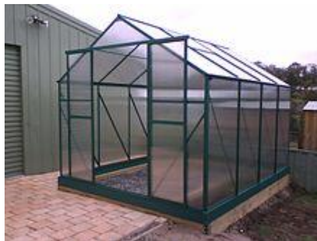
Polycarbonate sheeting in a greenhouse.
